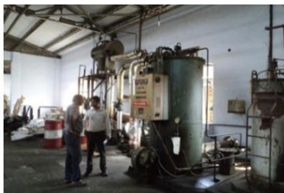
Thermax Make Diesel Boiler
